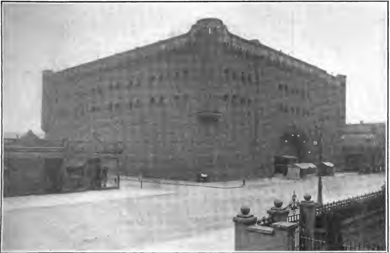
FIRST REGIMENT ARMORY, MICHIGAN AVENUE AND SIXTEENTH STREET, USED FOR OVERFLOW FROM COLISEUM SHOW.
